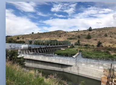
Outlet of Upper Klamath Lake/Link River Dam
