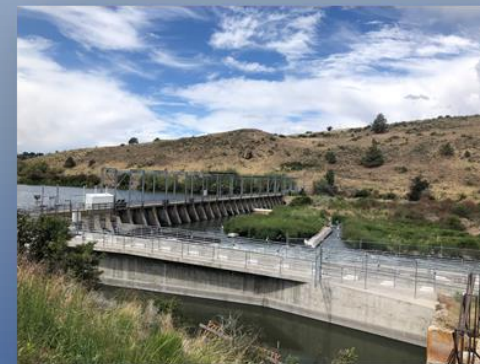
Outlet of Upper Klamath Lake/Link River Dam
