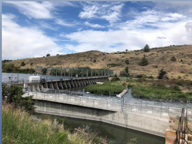
Link River Dam (outlet of UKL)
