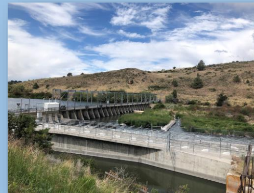
Outlet of Upper Klamath Lake/Link River Dam
