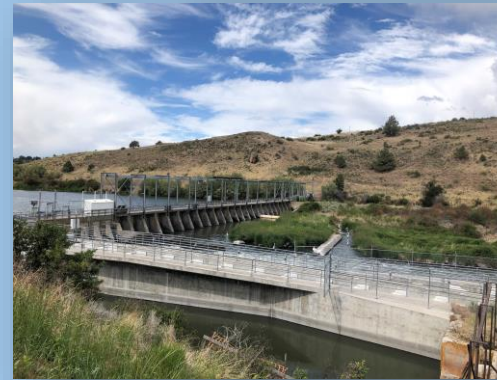
Link River Dam
